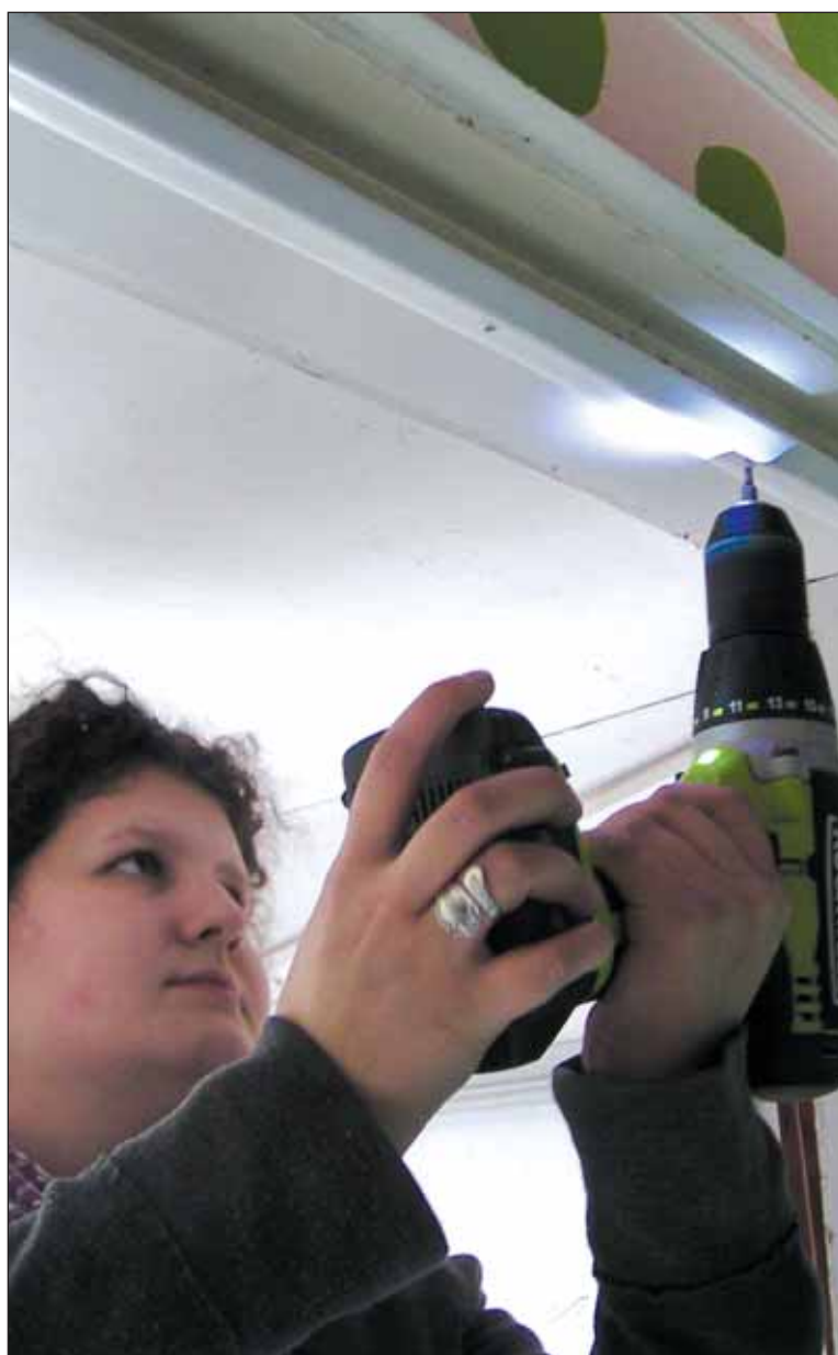
Daniel Butenhoff, a member of the Home Energy Squad, installs weather stripping around the back door of Erica Schumacher's Dudley Avenue house.
