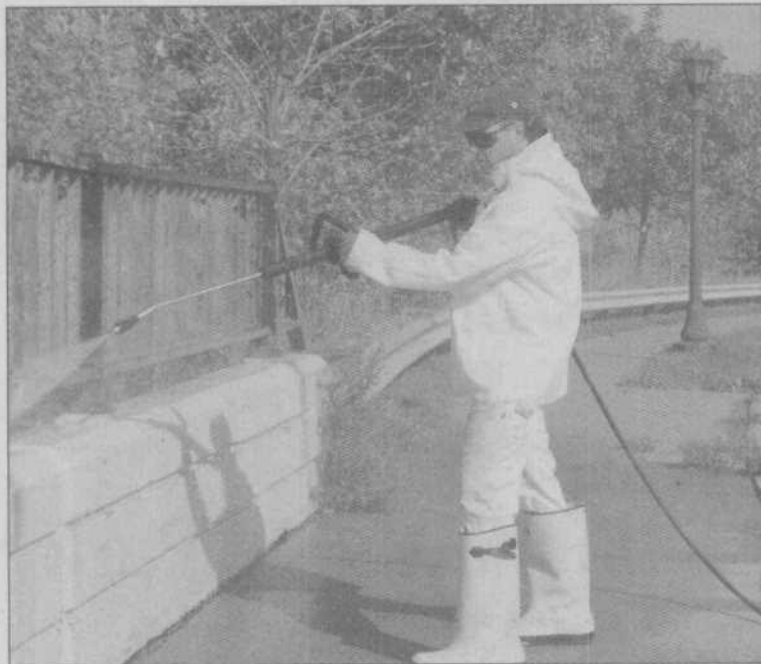
Department of Public Works employee Matt Stone removes loose paint from the railing of the Raymond Avenue bridge. The railing is being repainted, a project DPW hopes to finish before winter.
