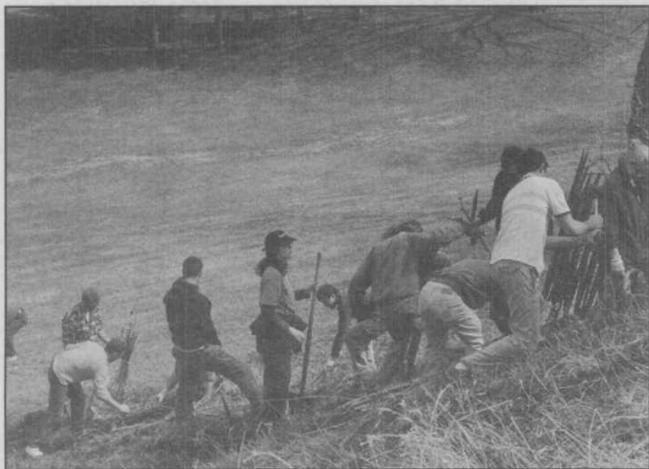
Landscape ecology students install erosion controls on the south slope of College Park. Photo by Ron Dufault
