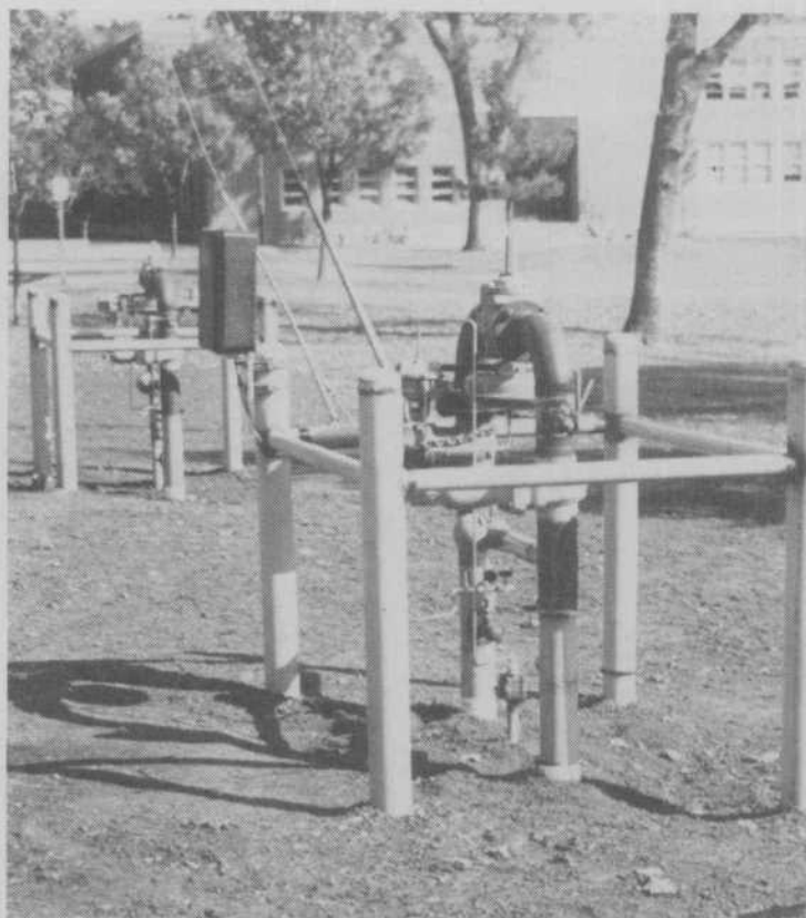
Photo by Laura Malchow, Central High School student NSP gas regulators have been installed recently at the north end of Langford Park, on the elementary school playground.
